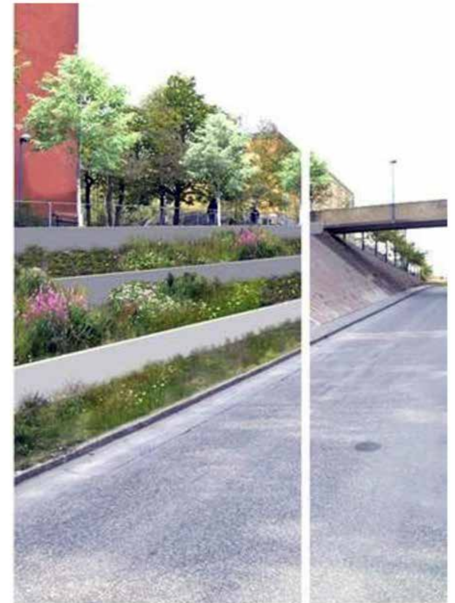
Figure 26. One example of a nature-based solution in a suburb in Stockholm. Instead of concrete slopes, a series of terraces have been proposed, filled with flowers. It will enhance both the aesthetics, lower temperatures, absorb heavy rains and promote biodiversity.
